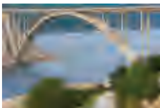
This bridge support arch is an inverted parabola.
