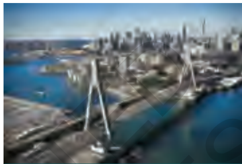
ANZAC Bridge in Sydney is a cable-stayed bridge in which each cable forms a triangle with the pylons and the bridge deck.
