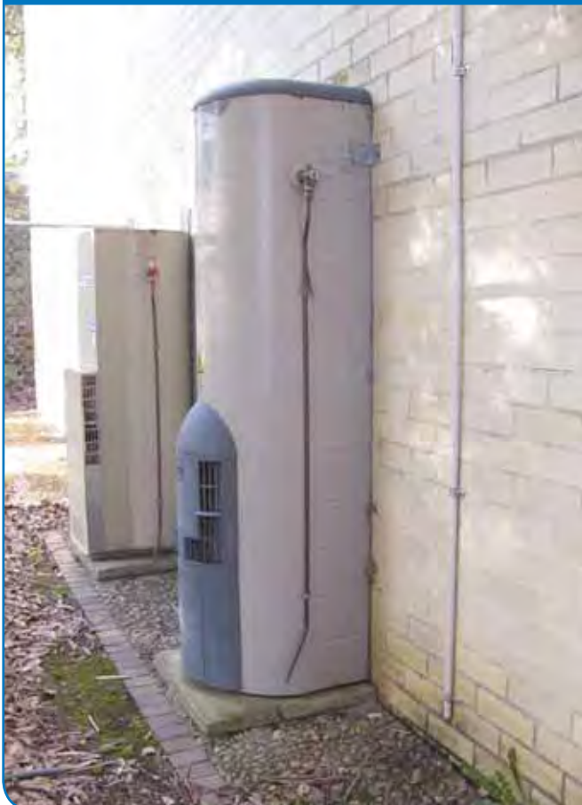
FIG 11.17 (a) Exterior fast recovery hot water services (foreground)
