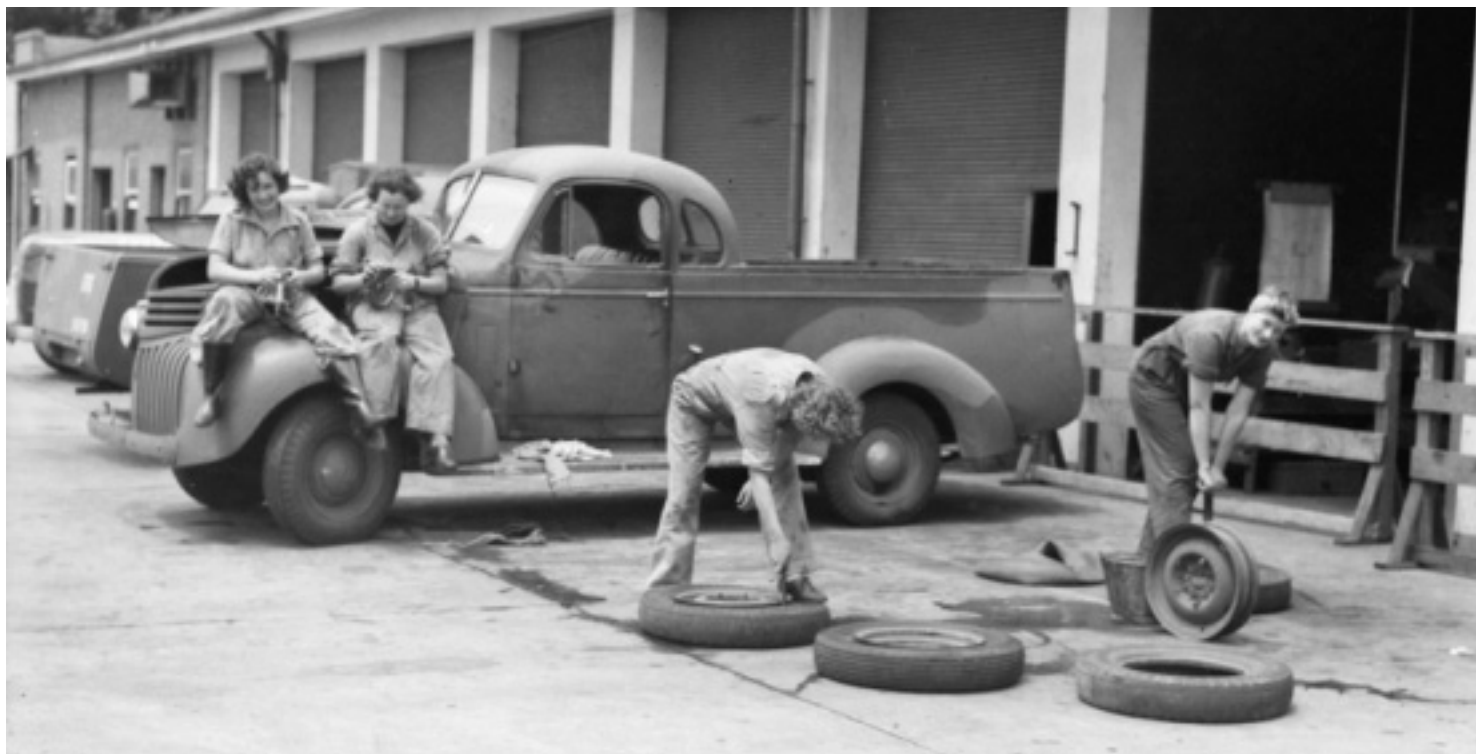
Source 2.93 Australian Women's Army Service mechanics carrying out maintenance work on Land Headquarters Signals motor vehicles at Albert Park, Melbourne (AWM 60917)
