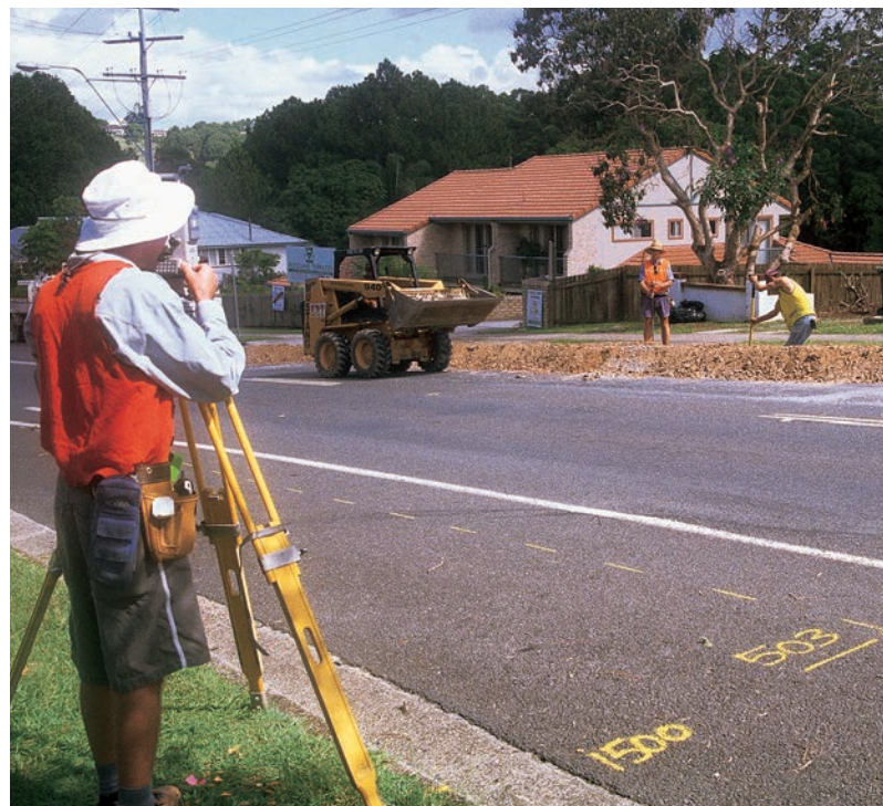
Fig 1 Surveyors use the property that light travels in straight lines to find the depth of the trench on the other side of the road.
